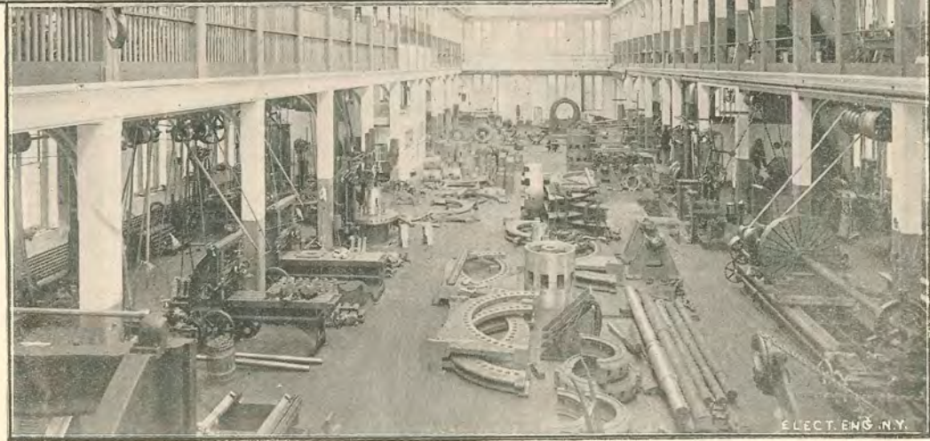
Interior Views of the Works on Kenne Avenue.
