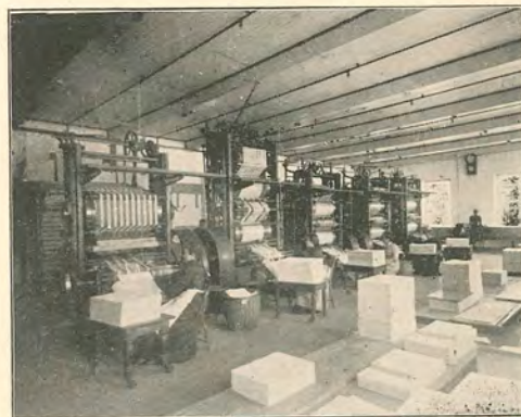
Finishing Room, Defiance Mill.
