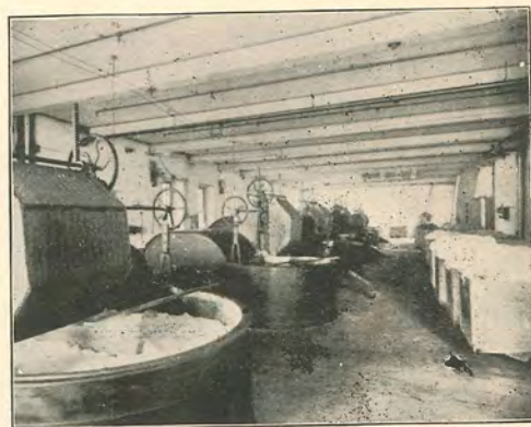
Engine Room, Defiance Mill.
