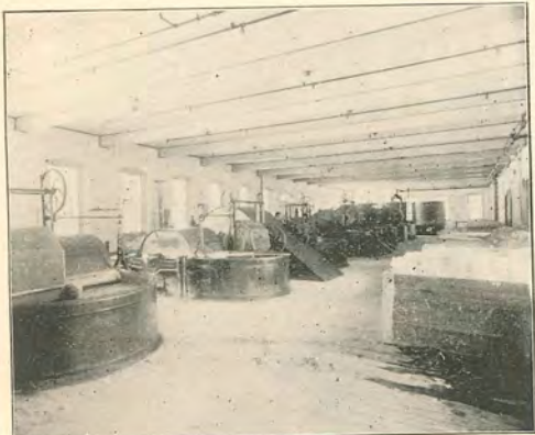
Engine Room, Centennial Mill.
