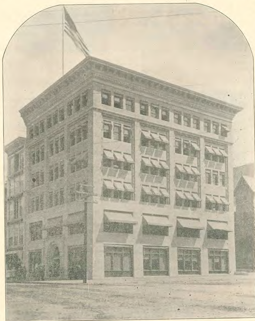
BERKSHIRE COUNTY SAVINGS BANK BUILDING.
