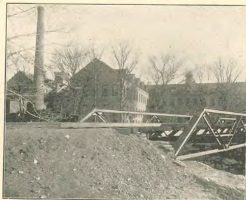
Rear View of Bay Sta'e Mill.
