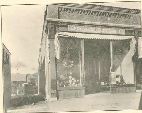
Berkshire Electric Company.
