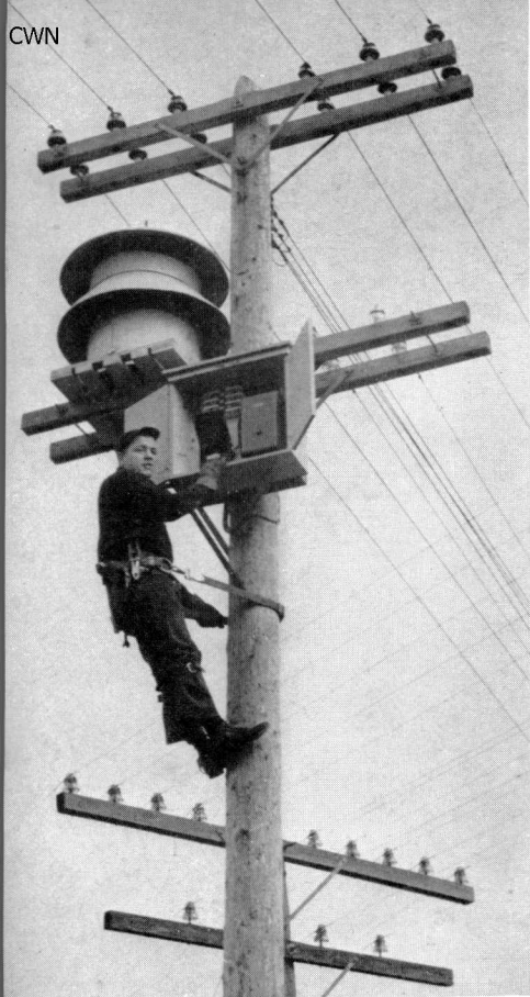
Lineman Warren Briggs checks one of the City's five electric air raid sirens.
